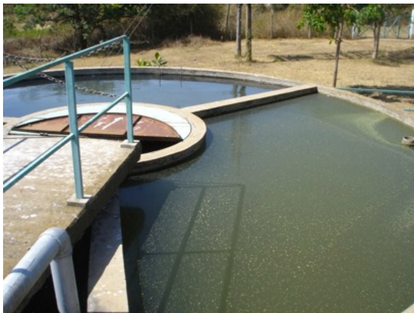
Figure 24. Coagulation tank showing algae growth on water surface
