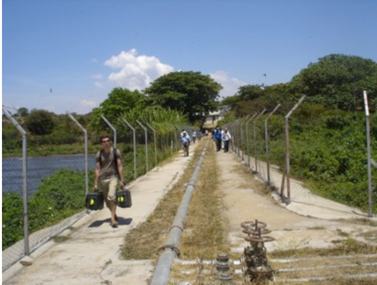
Figure 22. Pipes leading from intake to treatment plant
