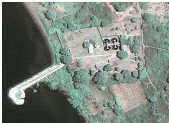
Figure 20. Lake Victoria water treatment plant
