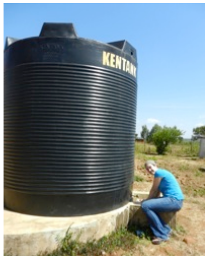
Figure 18. Storage tank collecting rainwater at Mabinju Dispensary
