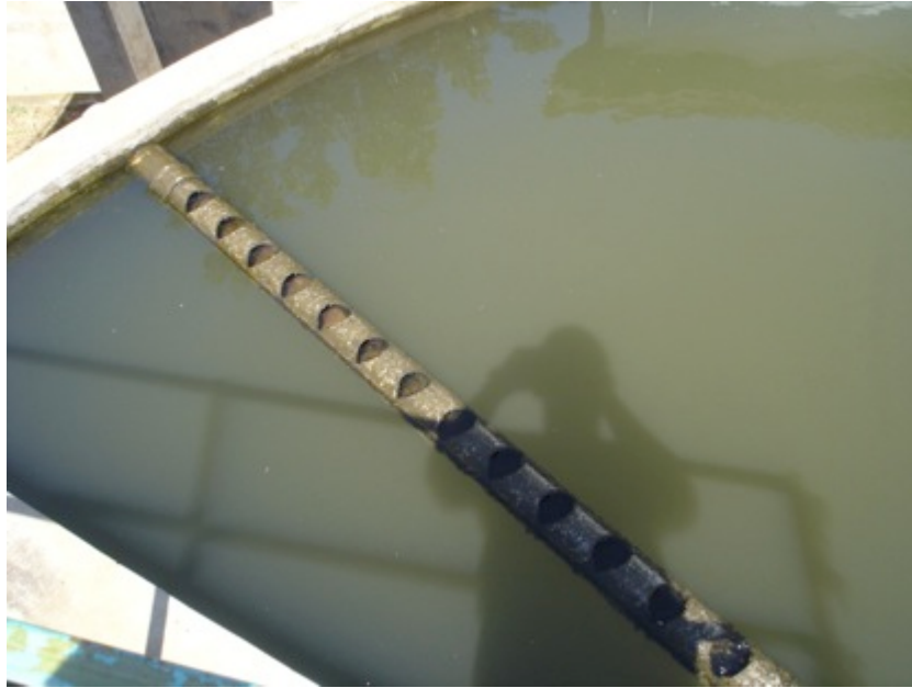
Figure 25. Pipe directing water from coagulation tank to filtration media
