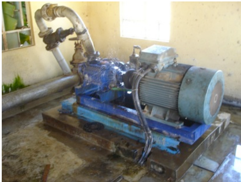
Figure 29. Leaky pump
