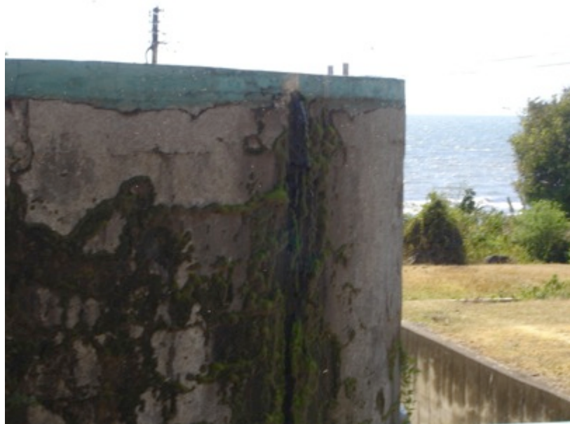
Figure 26. Side view showing leak in coagulation tank
