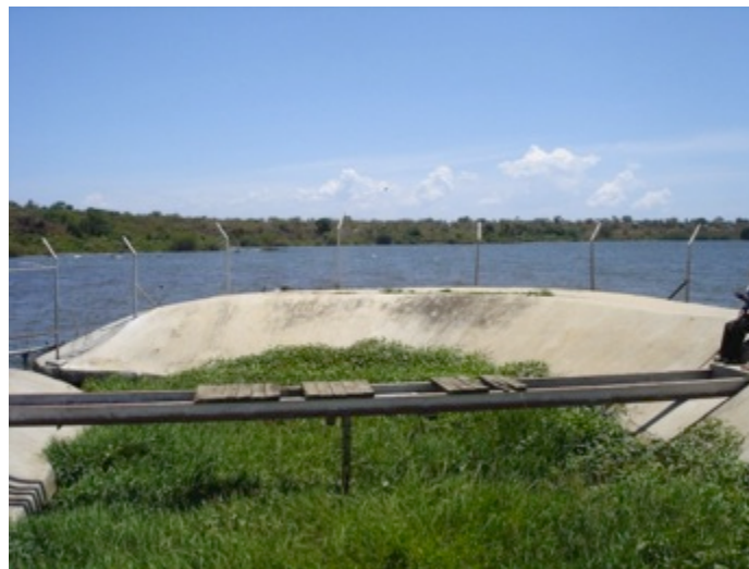
Figure 21. Concrete sump at treatment plant intake
