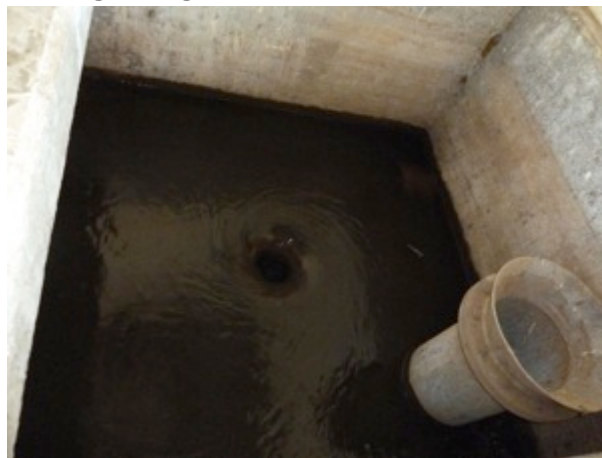
Figure 31. Mixing tank for potential coagulant application
