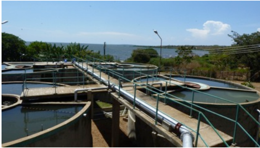
Figure 32. Coagulation basins
